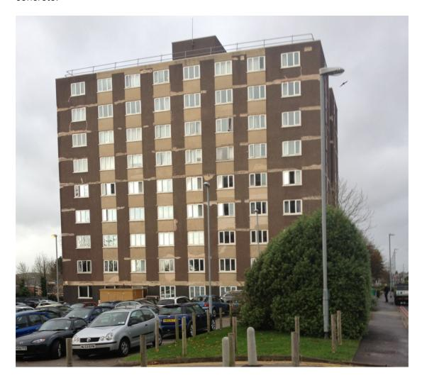
Ronacrete Approved Contractor Constructive Solutions carried out patch repairs to the concrete ring beams and to infill panels on the façade using RonaBond HB40 high build repair mortar. Ronafix Pre-packed Render/ Screed was used to provide a render finish to the concrete.
